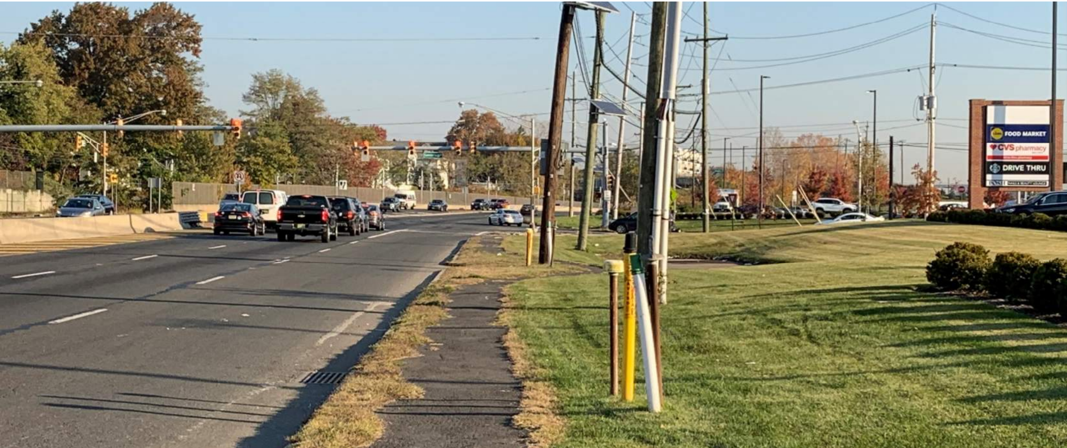
▶ Rt. 440 Northbound, Existing Asphalt Sidewalk, and Existing Utilities | Looking North
