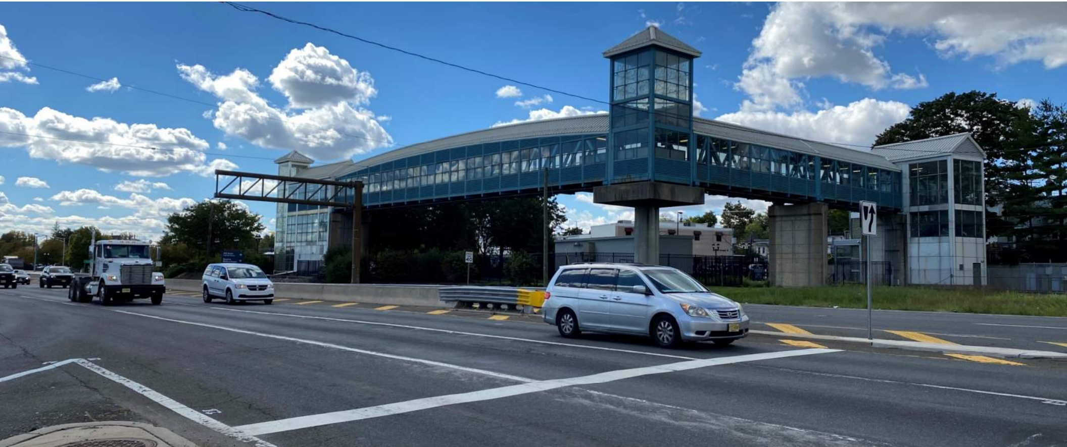
▶ Existing NJ Transit Pedestrian Facility from Goldsborough Dr. Intersection | Looking Southwest
