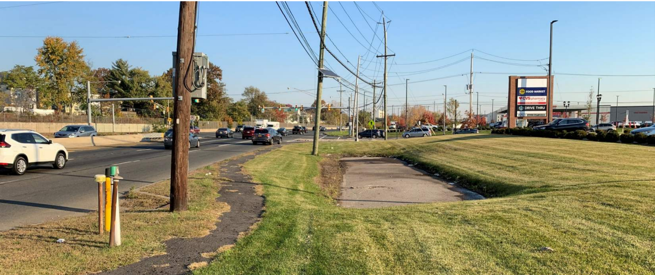
▶ Proposed East Landing Area and Existing Utilities Along Rt. 440 Northbound | Looking North
