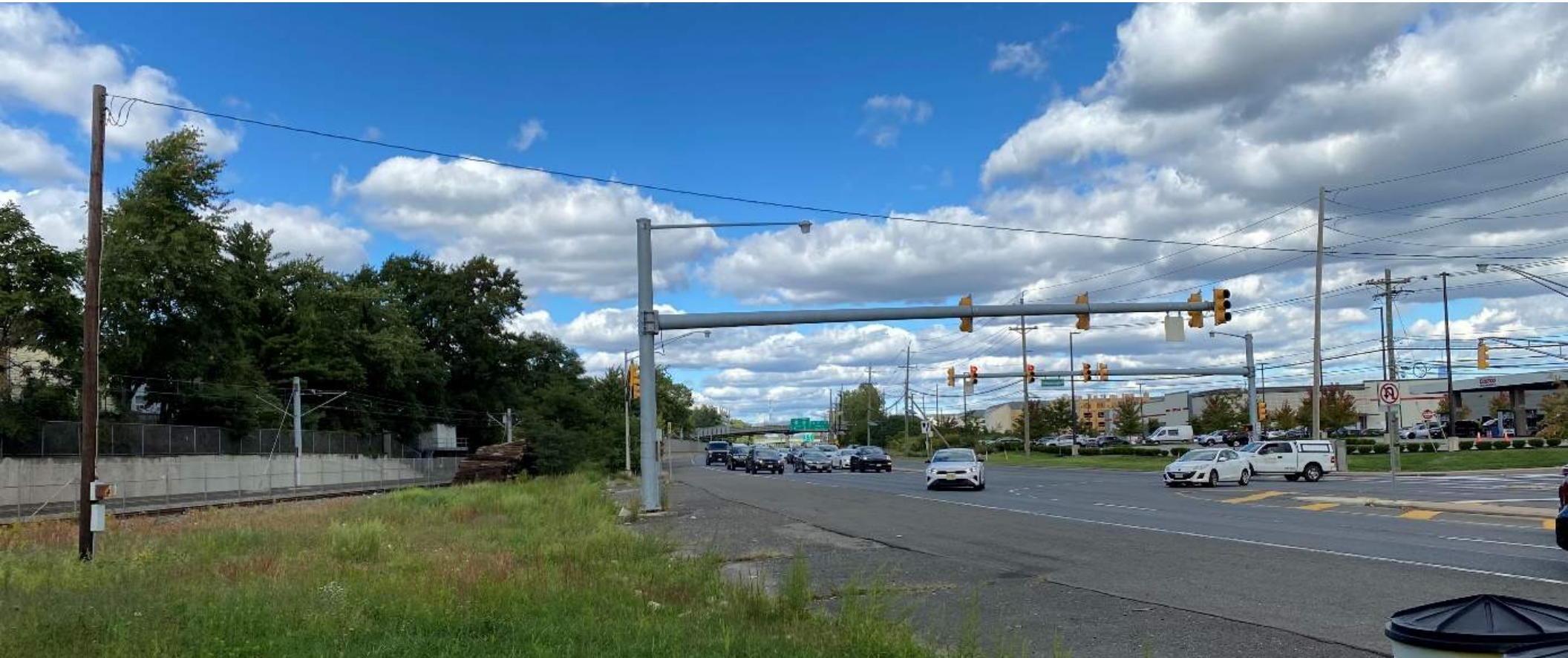
▶ Light Rail and Freight Railroad Tracks & Rt. 440/Goldsborough Dr. Intersection | Looking North
