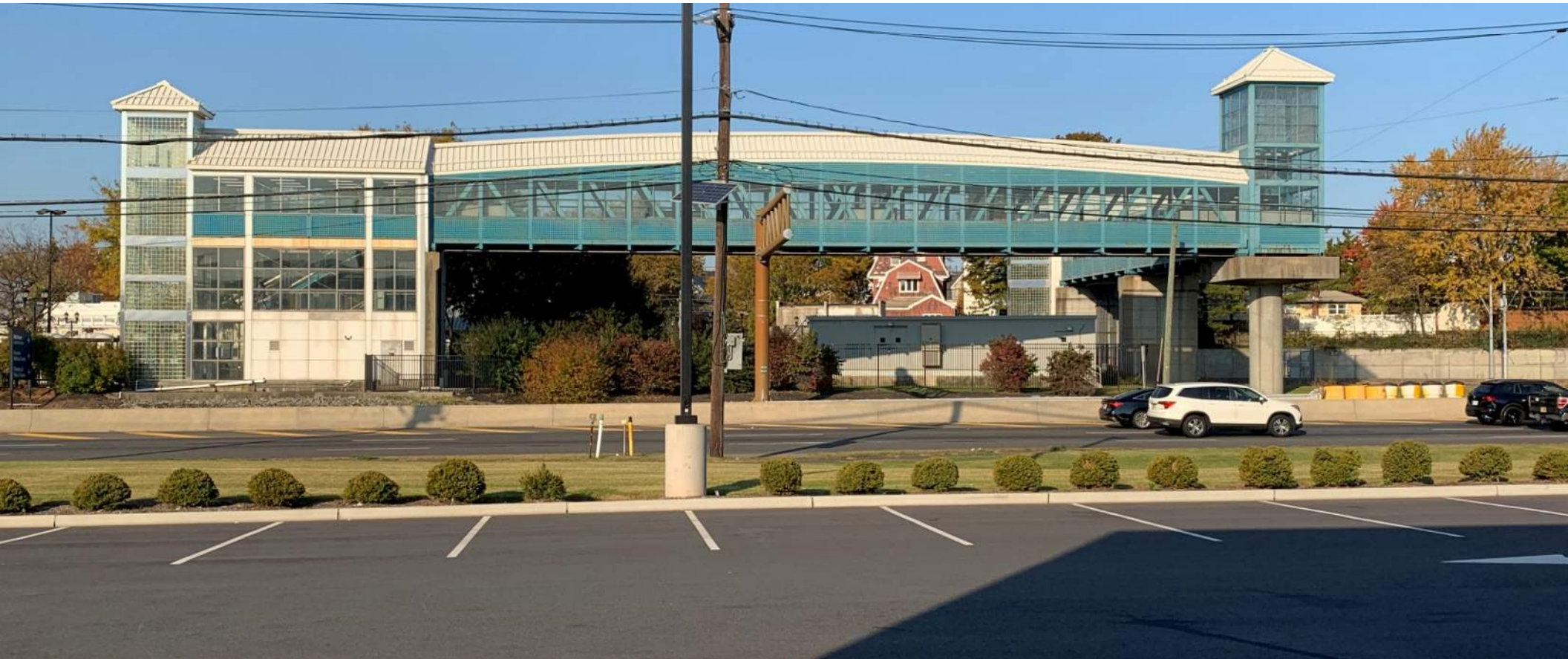
▶ Existing NJ Transit Pedestrian Facility from CVS Parking Lot | Looking West
