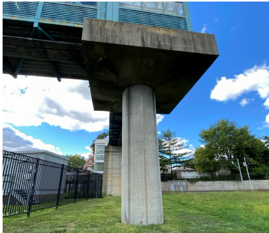
▶ Existing Pier at Tie-in Point | Looking West
