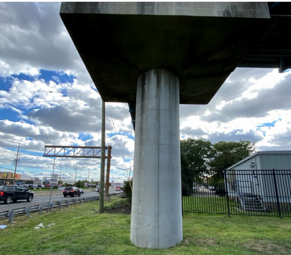
▶ Existing Pier at Tie-in Point | Looking South
