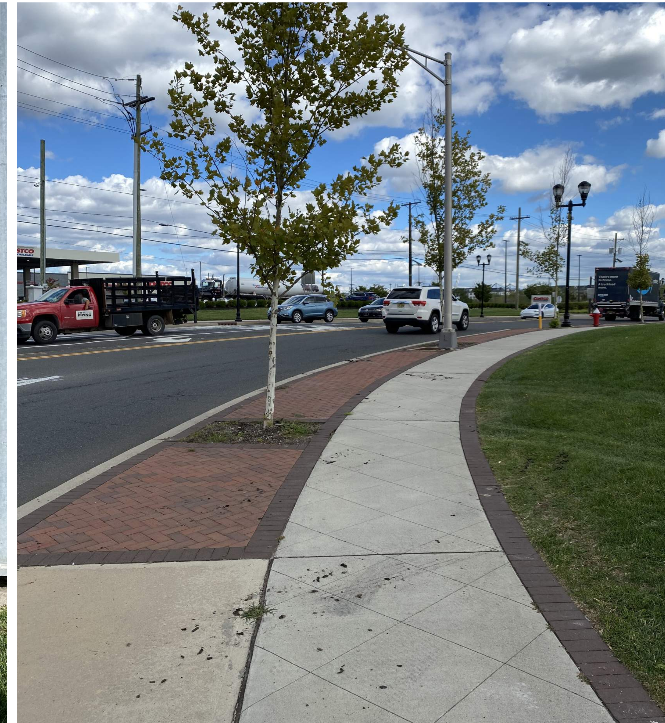
▶ Existing Streetscape Features Along Goldsborough Dr. | Looking East
